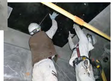
Installation of radioactivation-resistant epoxy resin boards at a leading-edge medical facility
