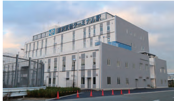
The Tokyo Cargo Terminal Station Office (Japan Freight Railway Company) designed and built by HAZAMA ANDO CORPORATION, utilized CFP and carbon offsets.
