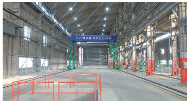
30-ton gantry crane.
