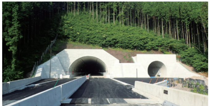
Completed shaft entrance.
