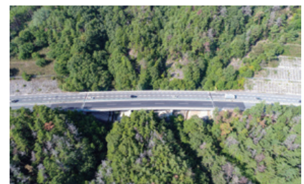
Kokuzo Bridge on the Nagano Expressway (new eastbound line is below).
