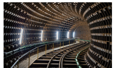
Curved section of the shield tunnel.
