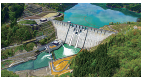
Tsugaru Dam (Aomori Prefecture) 2016
