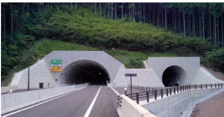
Futaenotoge Tunnel (Aso Block) (Kumamoto Prefecture) 2020 Japan's first new tunnel construction to use an early contractor involvement (ECI) approach, contributing to faster recovery after the Kumamoto earthquake. Excavation was completed in roughly half the typical period required. Received 2020 JSCE Outstanding Civil Engineering Achievement Award
