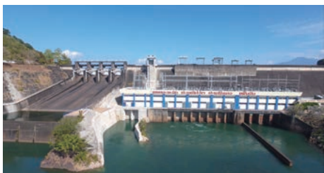
Nam Ngum 1 Hydroelectric Power Plant Expansion (Laos) 2022 This project entailed adding turbines to an existing dam built by our Company. Construction involved a high degree of difficulty, including building a new water intake by opening a hole in the existing dam, a first for Southeast Asia.
