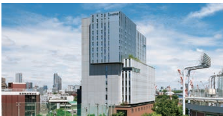
Nippon Seinen-Kan & JAPAN SPORT COUNCIL Administrative Building (Tokyo) 2017 This large-scale mixed-use complex, which includes a theater, hotel, and office space, used the lift-up method to lift mega truss structural components.
