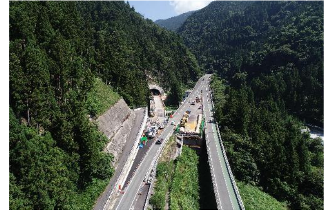
▲ San-En-Nanshin Aokuzure pass tunnel (tentative name) main construction
