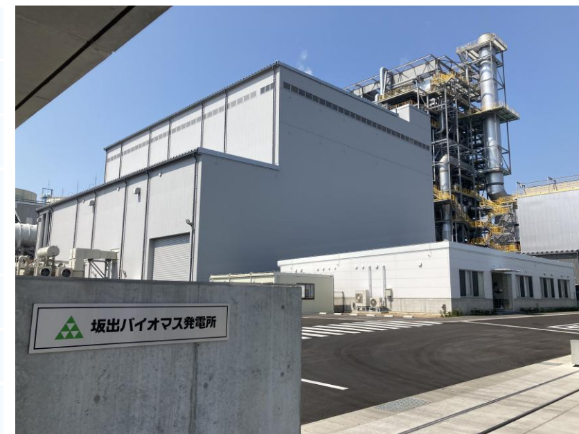
▲ Sakaide Biomass Power Plant
