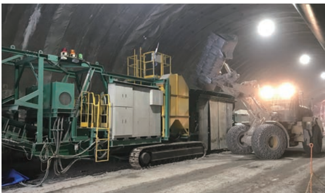
Mobile crusher (owned by Aoyama Kiko).
