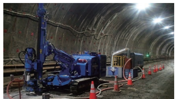
Trial construction in a tunnel.
