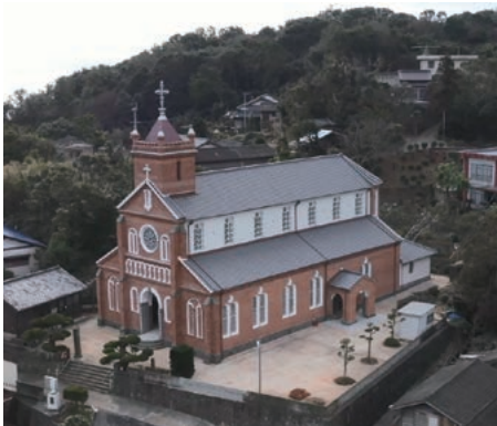
Kuroshima Catholic Church (photo provided by Sasebo City Board of Education).
