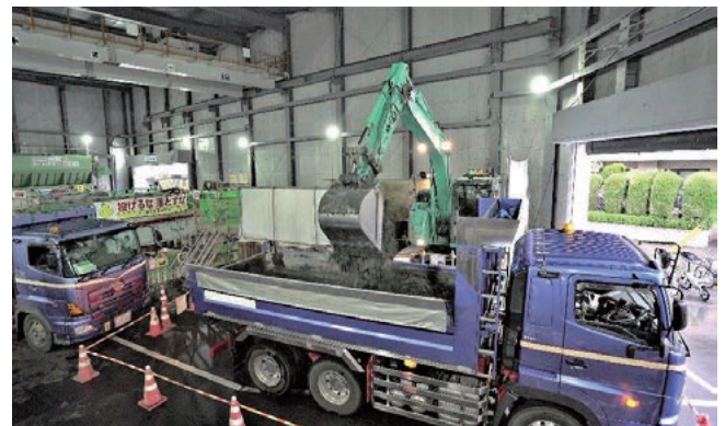
Trial autonomous operation of a power shovel.
