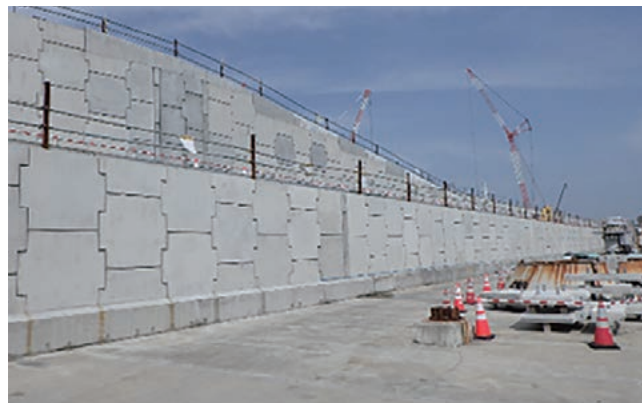
Part of the completed breakwater.
