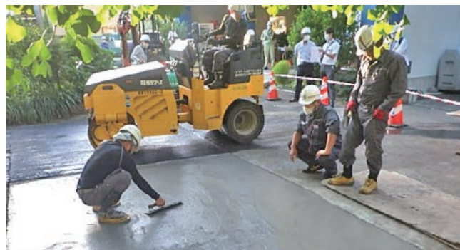
Construction trial using Carbon Pool concrete.
