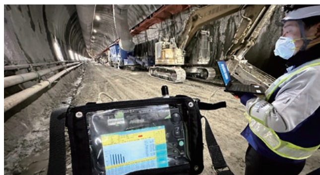
Trial at a tunnel work site.
