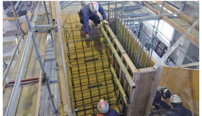
Full-size apartment staircase for training.
