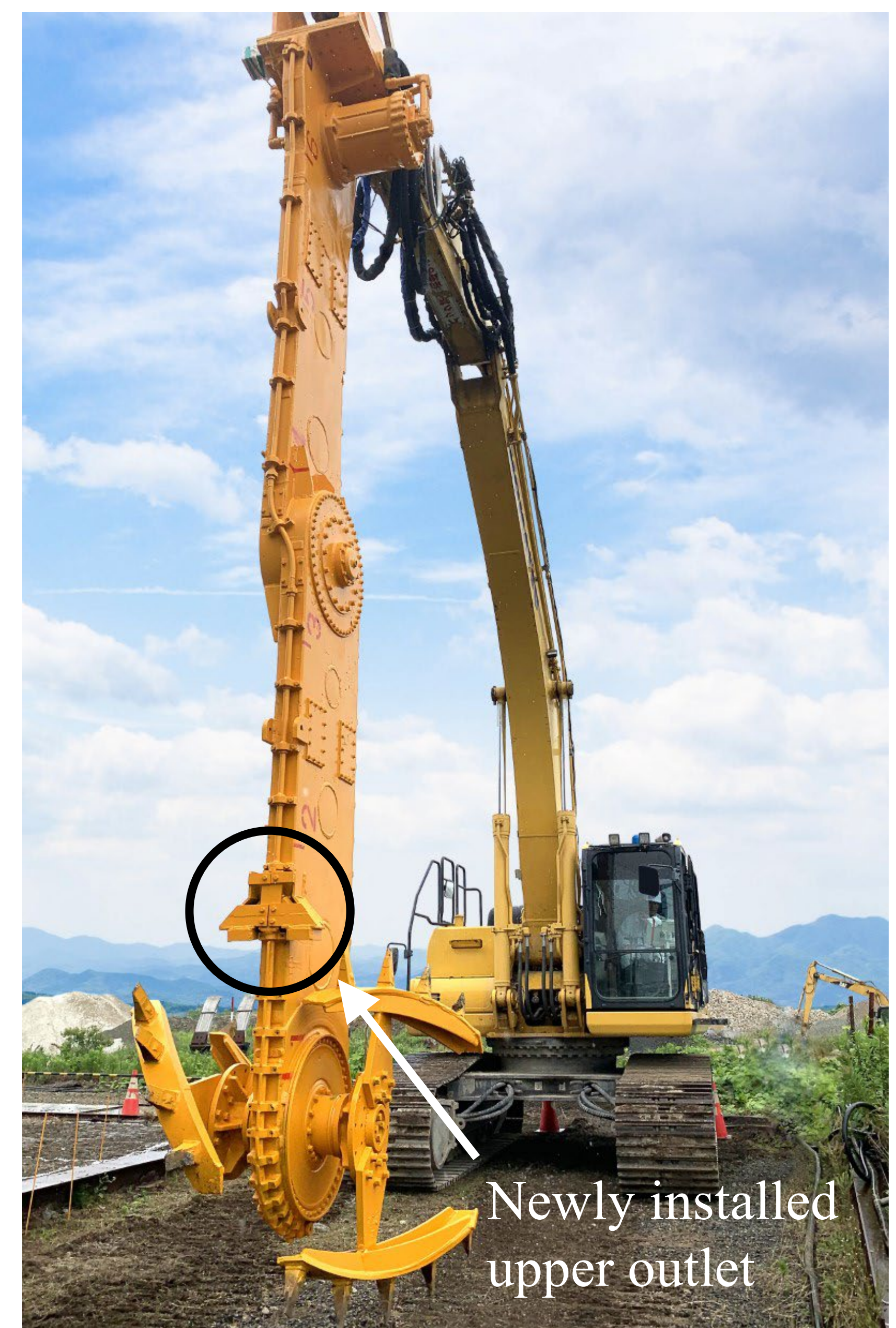
Construction machine of WILL-m method
