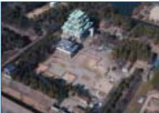
The central courtyard area is the site of the former Nagoya Castle Hommaru Palace.
