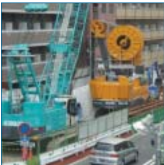
The Quattro Side Cutter in use at a construction site
